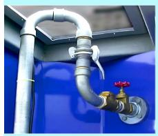
The guick release coupling on the pump galvanised discharge pipe allows the pump to be quickly removed from the chamber without any tools. This greatly cuts down servicing costs and should a pump need to be replaced, this again can be done with the minimum of disruption to the system.
